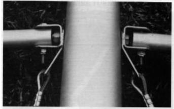
Photo 6 Spreader tube attachment
