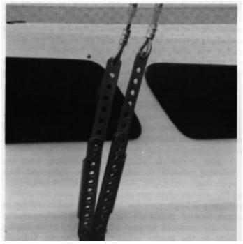
Photo 14 Wire adjuster channel attachments
