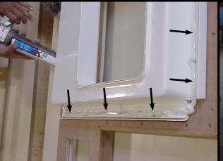
Secure the icebox top insulator to the bottom of the galley top using #10 x 1" flathead screws every 6" to 8". Caulk (using 5200) generously just inside the outside perimeter on the bottom of the icebox top insulator.
