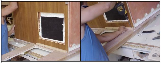
Before the foam that was placed between the icebox top and the icebox has had time to expand place the icebox face on the side of the icebox and secure it to the galley sub top.
