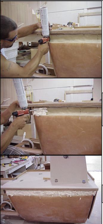
After filling the voids along the top on both sides apply expanding foam along the entire length of the cutout on the top back side
