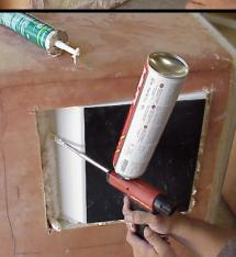
Also fill the voids between the insert and the icebox with expanding foam.
