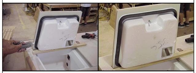
Caulk, using 733 white caulk, around the outside perimeter of the rubber gaskets where they meet the bottom of the icebox lid.
