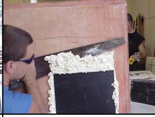
Using two people, flip the icebox up and place it over the icebox top insulator. Press the icebox down well to ensure a good seal then secure using #10 X 1-1/4" panhead screws. Secure every 6" to 8" all the way around box. Access "half circles" have been provided where necessary.
