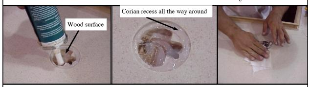
Before installing the handles on the icebox lids, fill cutout that will receive the handle with approximately 1/4" layer of 733 clear caulk. After the handles are installed clean up the excess caulk using alcohol. <u>CAUTION</u>: Avoid using acetone.
