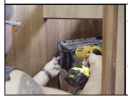
Place the insert cover over the insert and secure it to the wood face using #8 x 3/4 panhead screws every 4" to 6" around flange.
