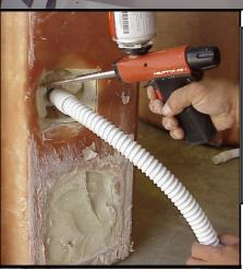
After attaching the drain hose to the bottom of the icebox with the proper size hose clamp, fill the cavity with expanding foam.
