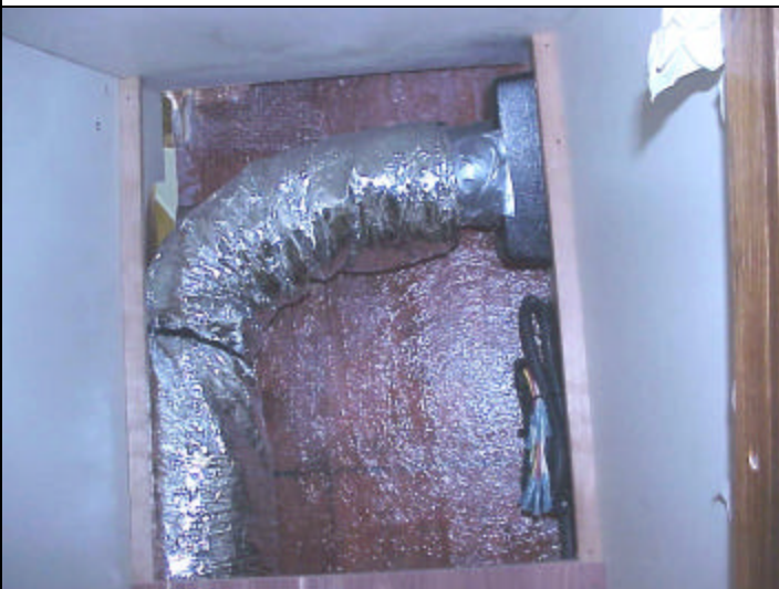
Flexible air duct to inside hanging locker to plastic grill box.
