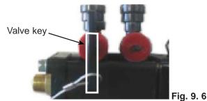
Shows the valve opened, notice the key is perpendicular to the line.
