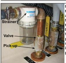
Image showing the intake valve and the strainer for the A/C system. Note the ball type valves. When the handle parallel to the supply line then it is in the open position.
