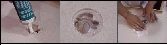
After removing the handle/latches on the icebox lids, fill the corian cutout with approximately 1/4" layer of 733 clear caulk. After the handles are installed clean up the excess caulk with a isopropyl alcohol.
