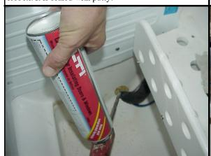
Foam the hole with expandable foam making sure all voids are filled. Be careful not to put to much foam in as the other side of the hole is open (next picture) and it might just keep running out of the hole.
