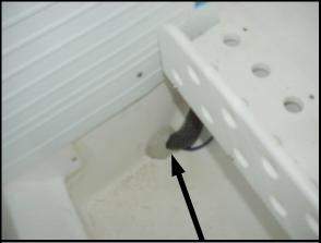
Refrigeration line comes into the icebox through the hole in the forward-bottom-outboard corner of the icebox. It is sealed with putty.
