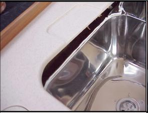
Apply a bead of 733 white caulk around the whole top of the sink lip then slide the back lip of the sink into the gap between the back hold angle and the bottom of the corian. After the sink has been tightly secured make sure that caulk squeezes out around the entire perimeter of the sink, add caulk if necessary. Clean up excess caulk using isopropyl alcohol.
