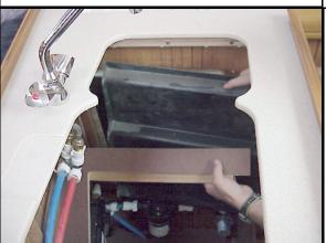
Lift the outboard end of the remaining shelf section up far enough to be able to remove the ABS cover. Remove the screws holding the cover on and remove the cover. Save the screws so they can be used to replace the cover later. There is one difficult screw to reach in the forward-lower corner of the cover (the water manifold is partly in the way), this screw will not need to be replaced as the shelf will hold the cover tight against the galley.
