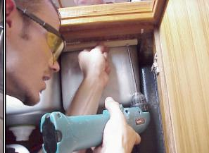
Attach the front holding angle to the galley plywood sub-top thru the pre-drilled holes using the #8 X 7/8" stainless steel panhead screws provided in the field kit. Make sure the sink is centered in the opening then tighten the back and front holding angle pieces.
