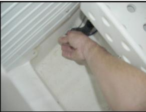
Remove the putty so the hole can be insulated with expandable foam.
