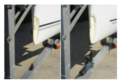
Using a utility knife, cut back to solid. Sand away the loose foam and taper plastic.
