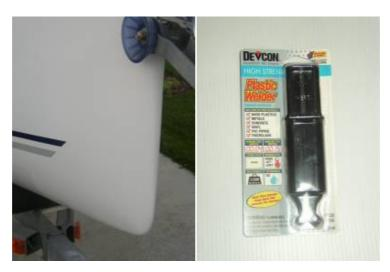
Repair is painted and polished the next day. This is the only place I very from factory recommendations, I use a two part urethane made by BASF, matched at the local automotive paint store. Plexus is sold under the name Devcon Plastic Welder.
