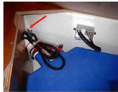
Lay out of: Tank
