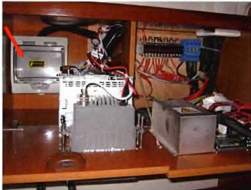
Decomposed switch 40A - Chart table unit
