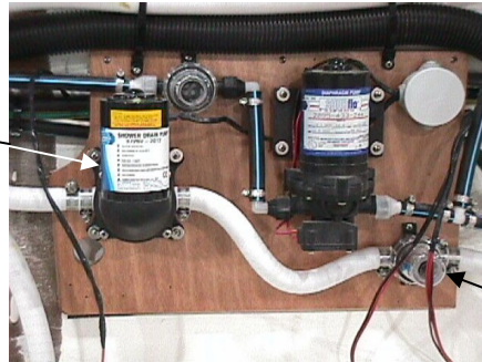
Plumbing Board – under sink in head
